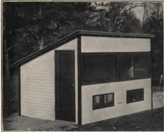
No. 3 LAYING HOUSE One Unit
